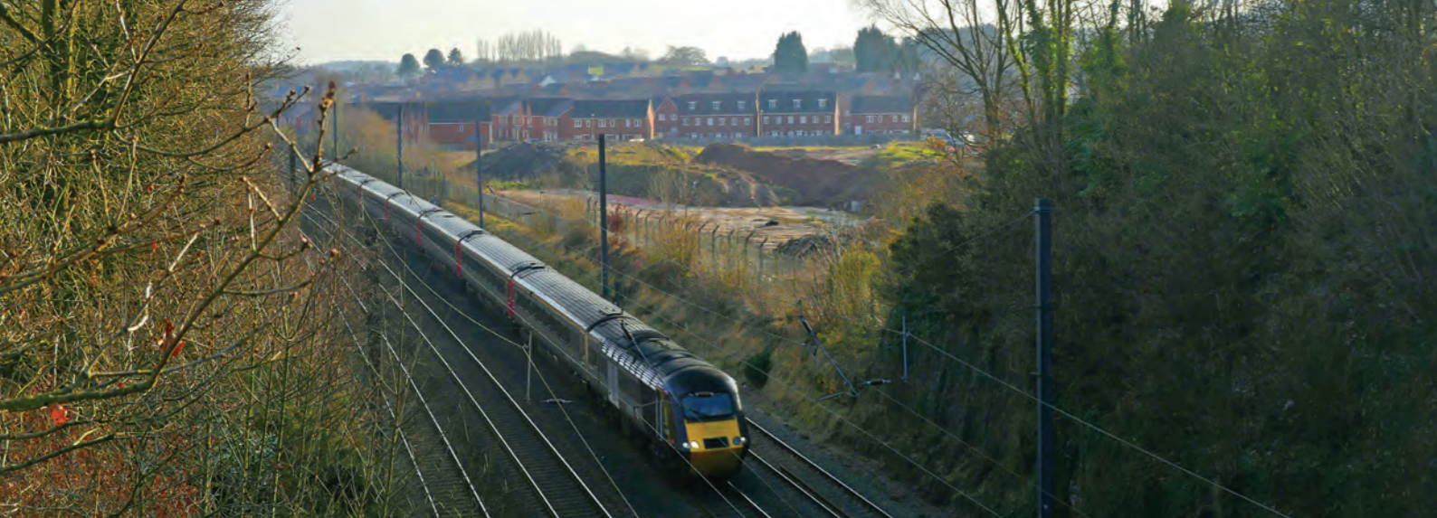
Railway line and new housing, Cofton Hackett
